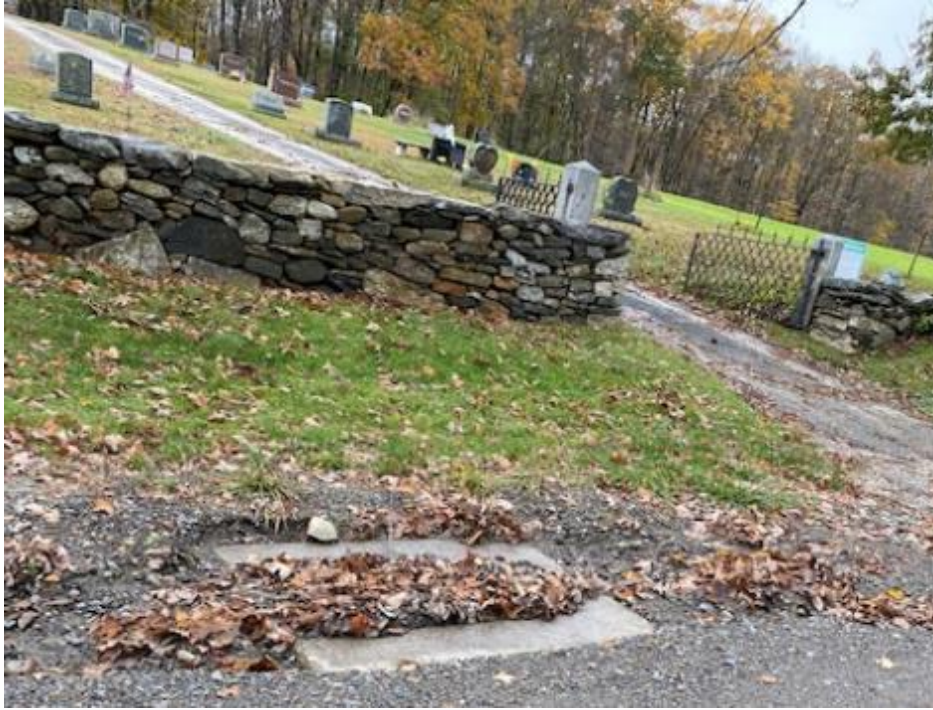
Figure 3 Existing storm drain on the south side of the cemetery entrance. It is clogged with a mixture of leaves and gravel after a recent rain event.
