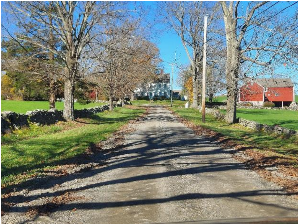
Figure 2 View of the tree line Center Cemetery Road from the County Road end. The cemetery is on the left side of this image. There is a gradual increase in elevation as you travel away from County Road. Note there are existing grass line swales on both sides of the roadway and gullies forming along both sides of the immediate roadway. Between the swales and gullies are piles of sand and gravel deposited by snowplows or the road grader. These piles act as berms preventing the stormwater runoff from sheeting off the roadway into the swales where the water would be slowed down and absorbed.
