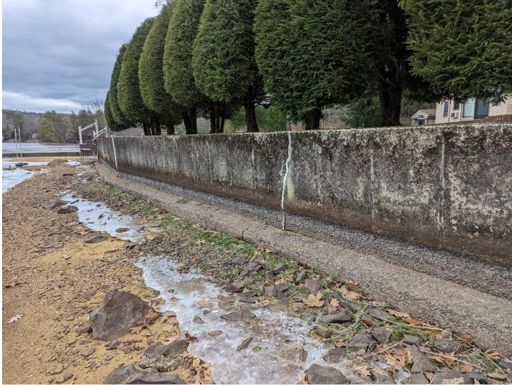
Image 1 – Poured Concrete Wall, Front View
