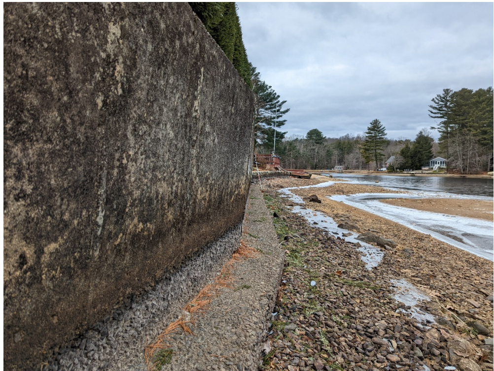
Image 2 – Poured Concrete Wall, Side View
