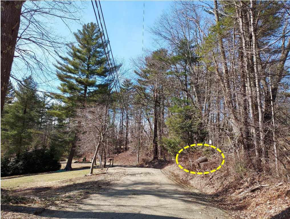
Photo 5 – The same viewpoint as noted in Photo 2, showing the tall trees noted in the previous narrative and the utility lines along the road. The circle area once again represents the seepage outflow area shown in the previous photos.
