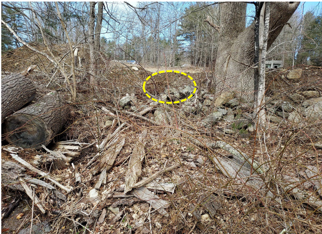
Photo 4 – The location of a small outlet pipe within the exposed soil berm atop the embankment.
