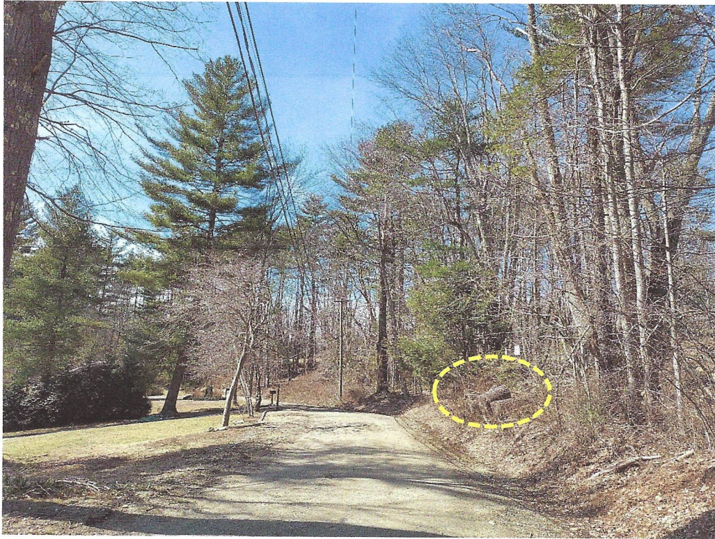
Photo 5 – The same viewpoint as noted in Photo 2, showing the tall trees noted in the previous narrative and the utility lines along the road. The circle area once again represents the seepage outflow area shown in the previous photos.
