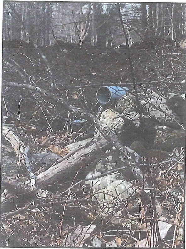
Photo 3: Outlet pipe from pond on Lake View
