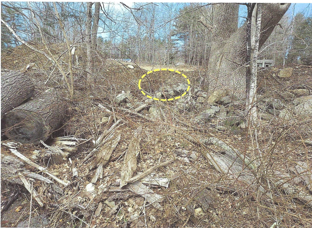
Photo 4 – The location of a small outlet pipe within the exposed soil berm atop the embankment.
